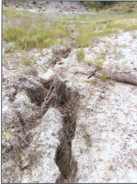
Photograph 9. Headward-migrating nickpoint in incised stream channel on western edge of ROW fill. View to southeast.
